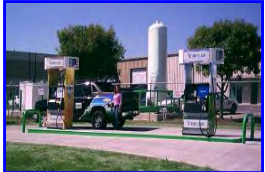
Bexar County Fleet fueling site in Texas
